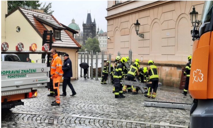
Flood Defence being erected by firemen in mid-September
